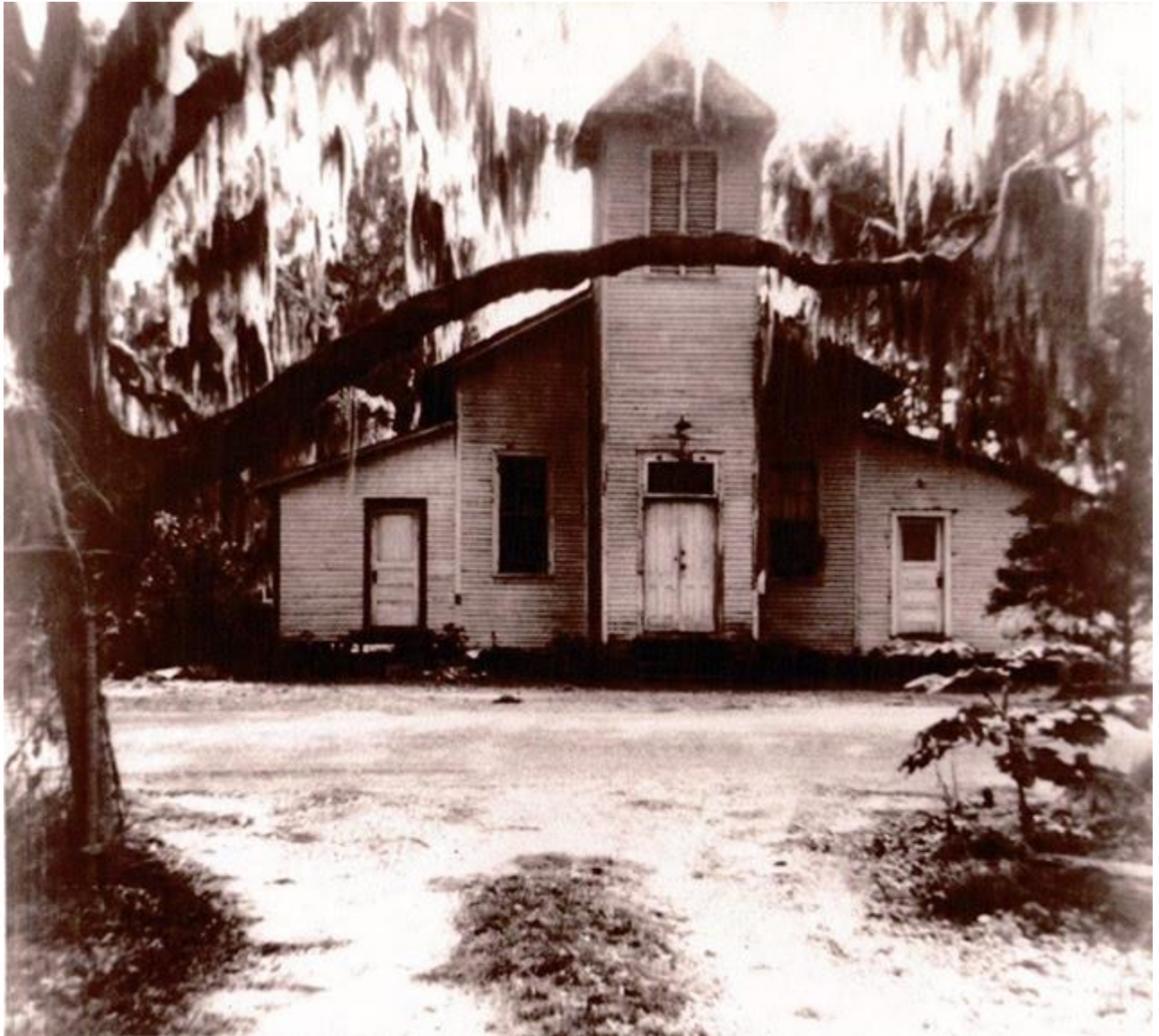
THE MANDARIN COMMUNITY CLUB, CIRCA 1953, NOT LONG AFTER RELOCATION TO ITS CURRENT SITE. THE BUILDING WAS MOVED FROM ITS PERCH NEAR THE ROAD ABOUT 100 FEET SOUTHWEST. AFTER THE MOVE, THE BASEMENT AND STAGE WERE ADDED.
